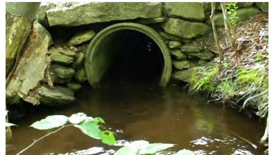
Figure NR10 - An undersized culvert in North Hampton shows evidence of being too small causing erosion on the stream bottom and banks. Photo: RPC staff.
