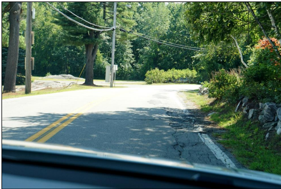
Figure 4. Wentworth Road near Shaw Circle showing section of ledge constraint, limiting expansion potential to proposed two feet
