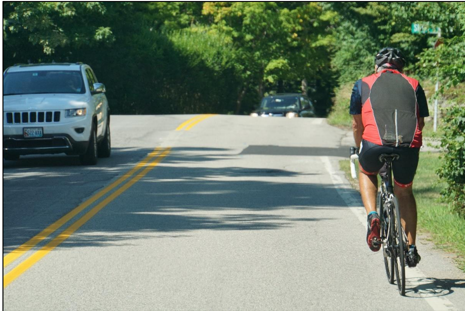
Figure 1. Person bicycling in travel lane due to lack of space right of fog line
